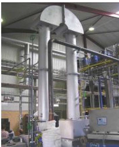
Figure 7. Test installation of Pilot-scale GSC test.
