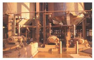
The average underflow rate from a decanter is typically 35% of the feed flow rate. The recirculation rate is maintained at approximately half of the underflow rate. As can be seen from the picture above, the underflow and recirculation flows exit the decanter through the same 8-inch outlet. This has been a problem because the underflow pump and the recirculation pump tend to compete for flow from the decanter. A great majority of time the underflow pump was at maximum output.
