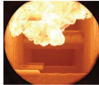
Figure 1 Turbulent diffusion flame inside a flue wall
