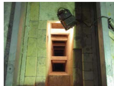
Figure 3 Testing unit refractory wall under assembly
