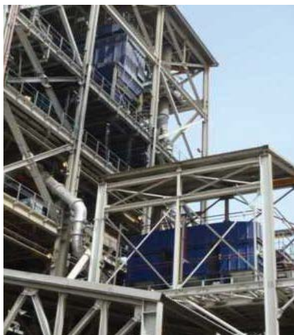
Figure 1: Eolios at Qatalum paste plant
