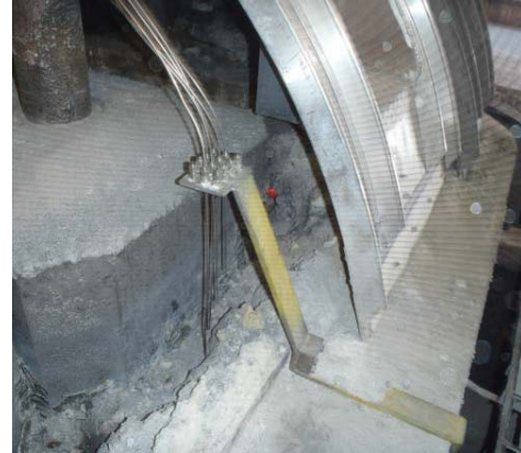
Figure 7. Thermocouples assembly inside the industrial electrolysis cell
