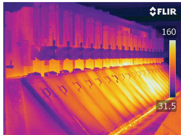
Figure 5. Thermal imaging of reduction cell showing variation of anode rod temperature across the cell.
