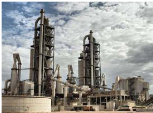
Figure 5. Picture of a cement plant with preheater and calciner kiln system.
