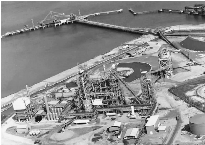
Figure 2.3 The CAL Circored facility in Point Lisas, Trinidad
