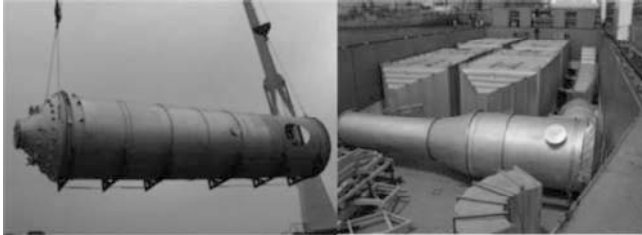
Figure 6. Modular Design Left Photo – Fully Fabricated Cooling Tower Right Photo – Preassembled Baghouse and Stack Section
