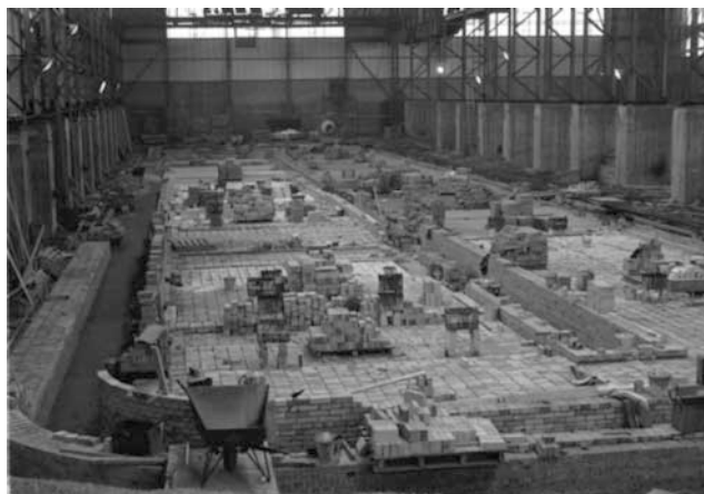
Figure 1. Construction site of the Riedhammer furnaces #1 and #2 in Årdal (1958).
