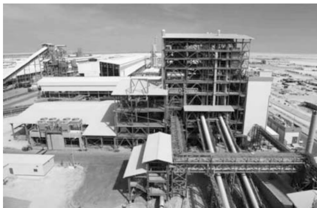
Fig. 1: Green Anode Plant at EMAL
