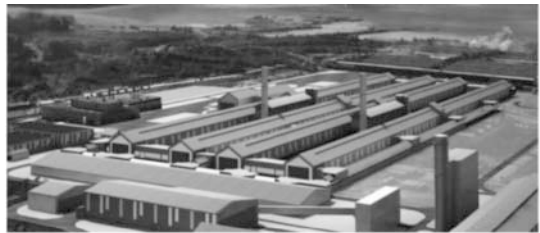
RTA plant bird's eye view
