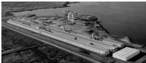
RTA plant bird's eye view
