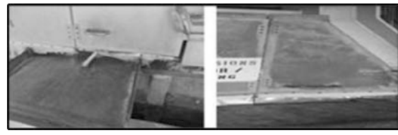
Figure 15: Fixing a light aluminium sheet at the bottom of cell door
