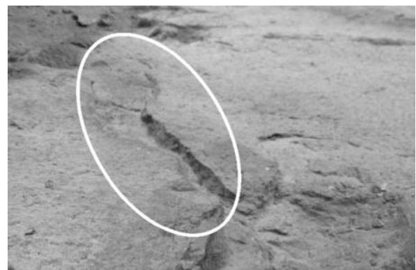
Figure 7. Shallow cracks on the cathode block surface after metal pad extraction, going 1-3 cm inside cathode panel
