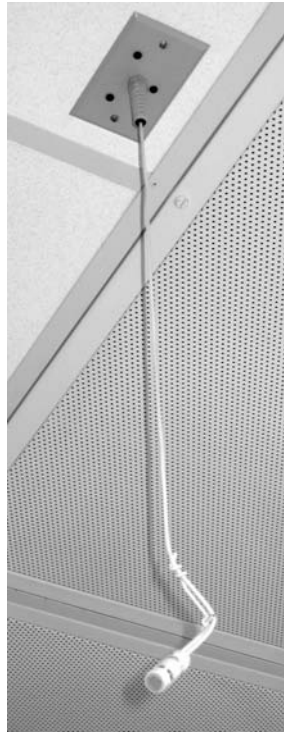
FIGURE 14.3 A ceiling-mounted microphone.
