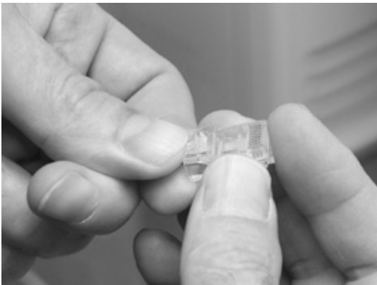
Figure 22-25 Inserting the individual strands
