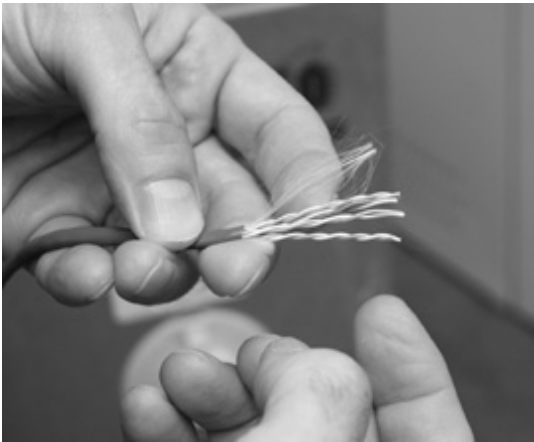
Figure 22-24 Properly stripped cable
