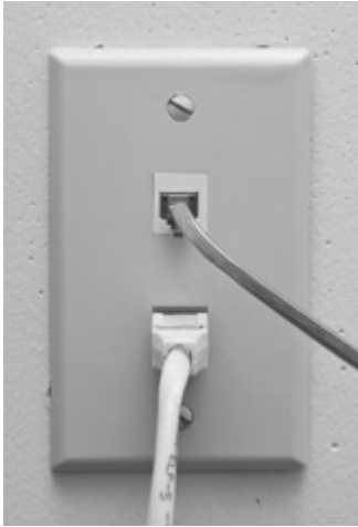
Figure 22-30 Typical work area outlet
