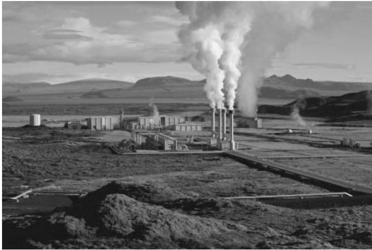
Figure 13.7 The Nesjavellir geothermal power plant in Iceland (Source: http://en.wikipedia.org/wiki/Nesjavellir_Geothermal_Power_Station )
