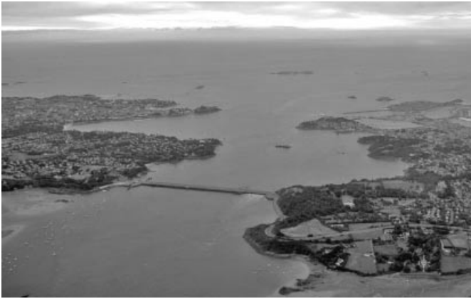
Figure 13.4 Aerial view of the Rance Tidal Barrier and generating station (Source: http://en.wikipedia.org/wiki/Rance_Tidal_Power_Station )
