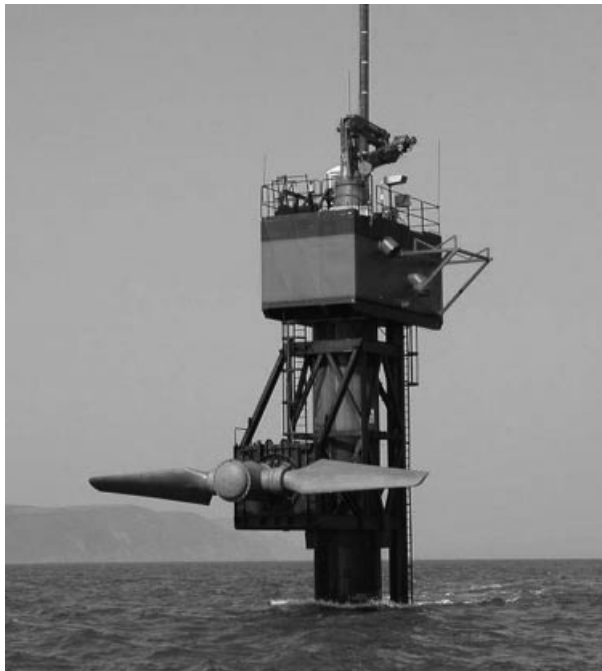
Figure 13.6 SeaFlow with its rotors raised (Source: http://en.wikipedia.org/wiki/Marine_Current_Turbines )
