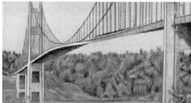
Figure 5.34. Illustration of Deformation of a Bridge Deck - Tacoma Bridge
