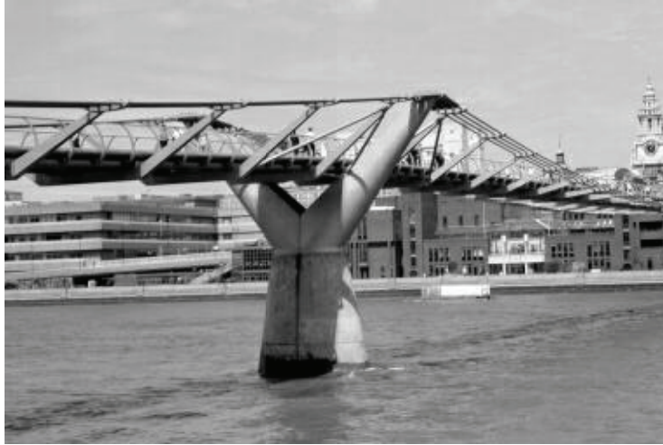
Figure 5.27. Millenium Bridge in London
