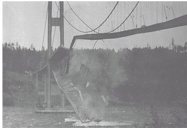
Figure 1.1. Tacoma Narrows Bridge Destruction
